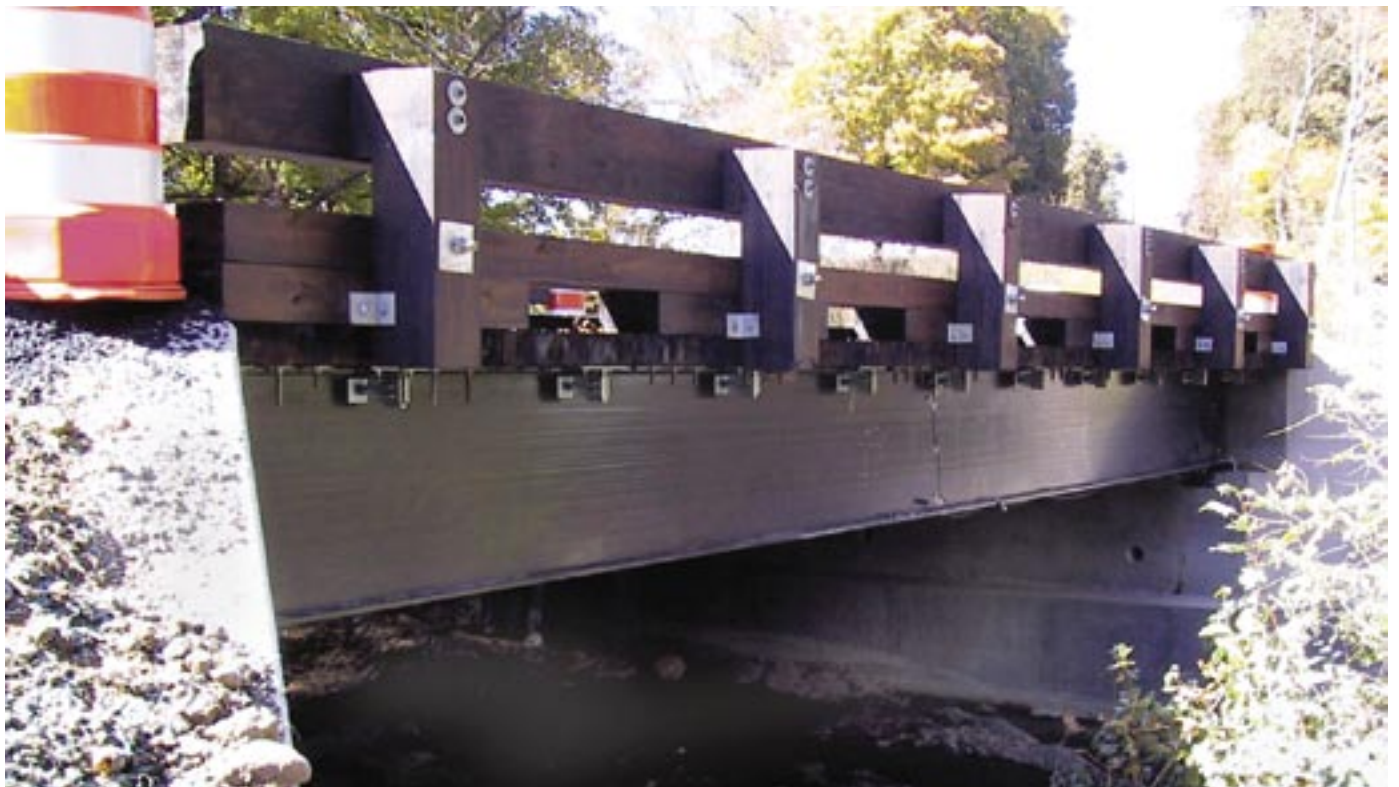
The Virginia Department of Transportation chose the 36" x 18" EXTREN DWB® to construct a 38' bridge in Sugar Grove, Virginia.
